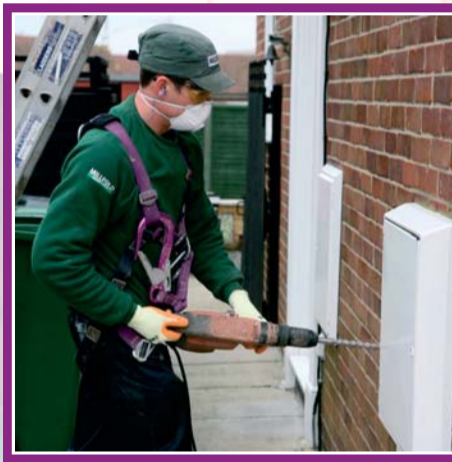
Access holes are drilled.
