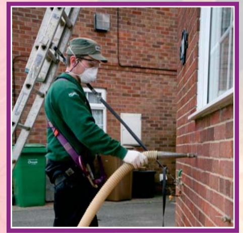
Your chosen insulation material is pumped into the drilled holes.
