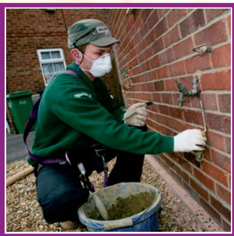
The holes are refilled.
