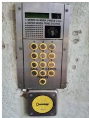
The electronic locks should “fail safe”, so that the locks release automatically in the event of total power failure to the locks.
