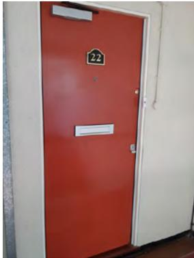
As discussed above, it is accepted that, in older blocks, fire doors, particularly flat entrance doors, do not meet current test standards for FD30S doors. However, these doors may still be acceptable if the doors remain in good condition, and they met the relevant standards at the time of construction of the block.
