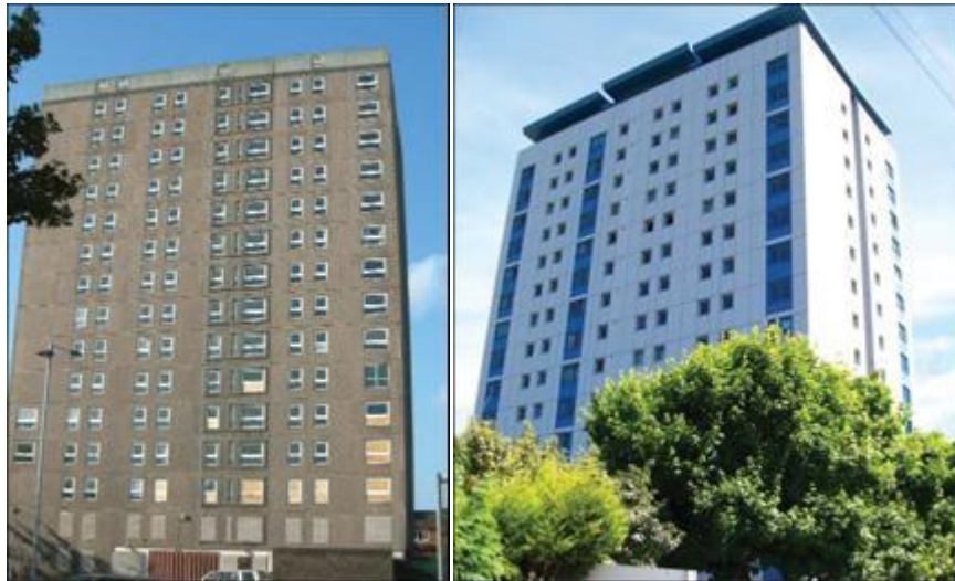
Figure 4.2: Before and after images of large scale high-rise refurbishment in the UK (D & B Facades, 2008)
